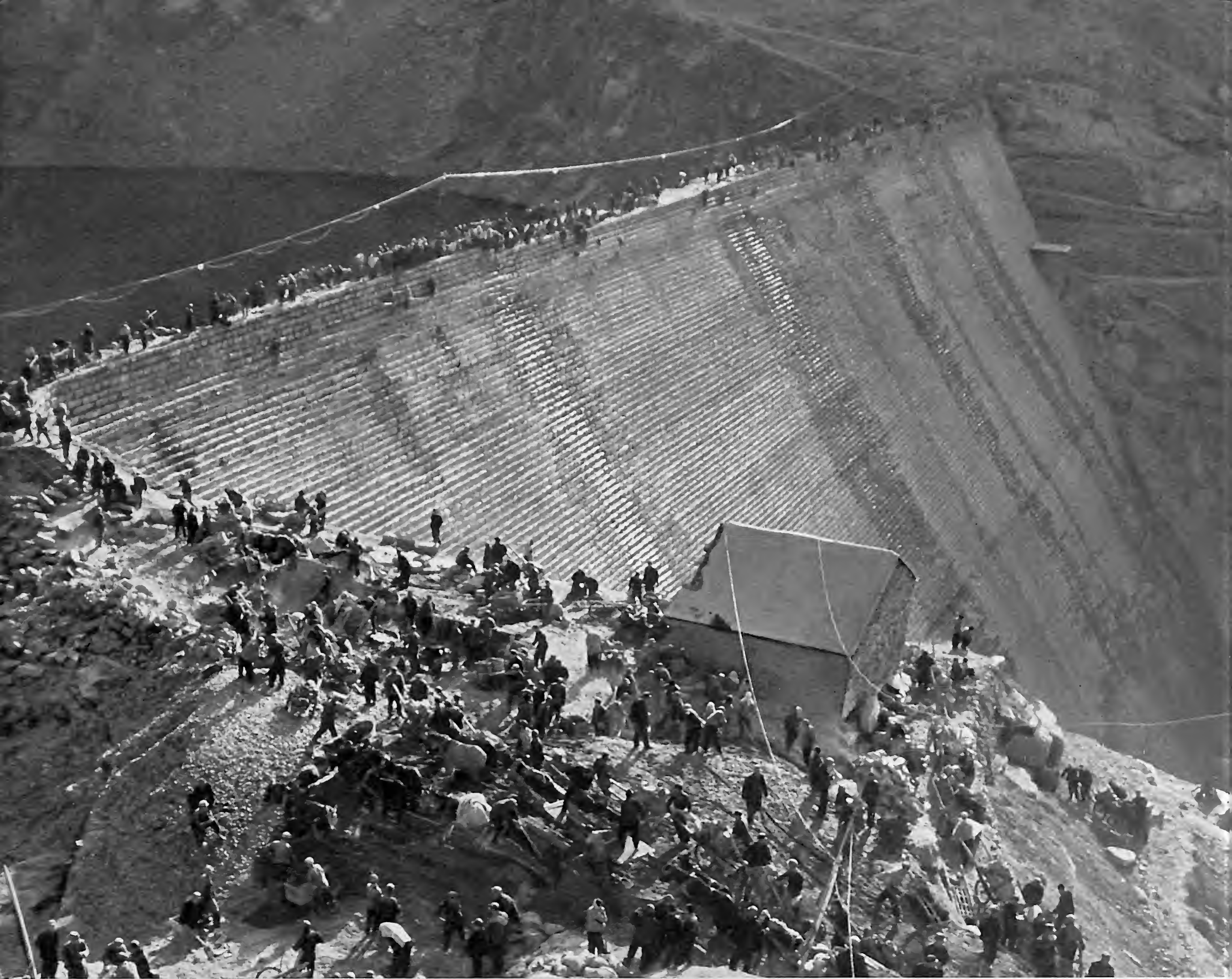
Constructing a reservoir.
